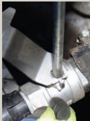
Installation Kugelhahngriff
